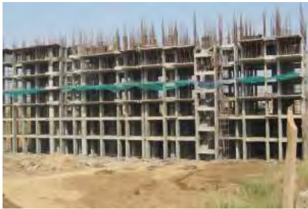
Navodaya - construction photograph
